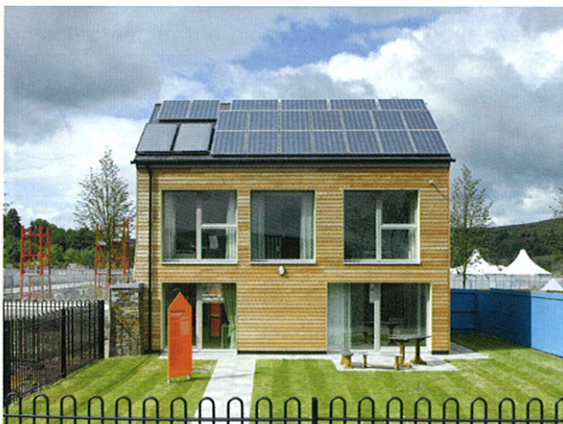
The Larch House, (left) and Lime House (right) still under construction.
