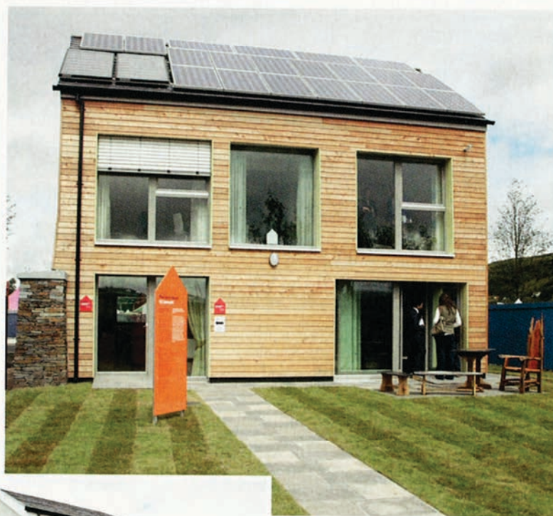
Ebbw Vale PassivHouses: three-bedroom Larch House (above) is clad with Welsh larch. Two-bedroom Dragonboard House (left) is clad with Welsh lime render
