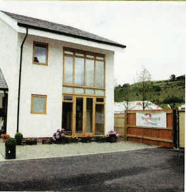
Ebbw Vale PassivHouses: three-bedroom Larch House (above) is clad with Welsh larch. Two-bedroom Dragonboard House (left) is clad with Welsh lime render
